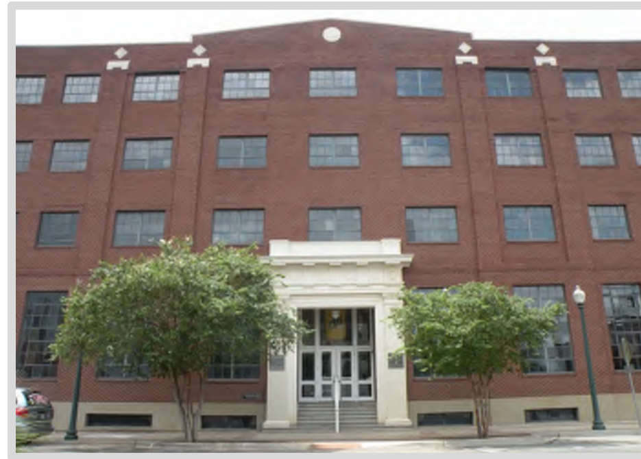
Image 7.11: Insurers of Texas Building, an example of adaptive reuse of a warehouse as office and historic preservation using national and local incentives
