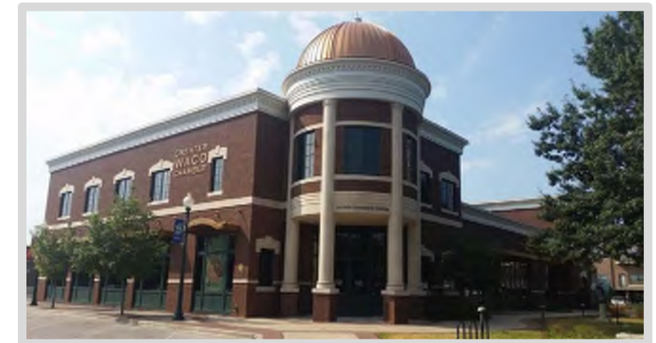
Image 8.3: The Greater Waco Chamber of Commerce built America's First Green Chamber of Commerce building in 2008, and has received a LEED (Leadership in Energy and Environmental Design) certification at the gold level for its headquarters and regional marketing center at 101 S. Third St. at Heritage Square
