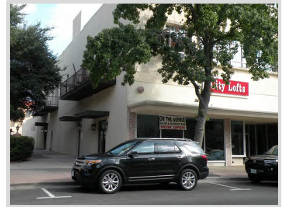
Image 7.9: City Lofts at the 700 block of Austin Avenue, showing a mixed use building abutting a landscaped sidewalk
