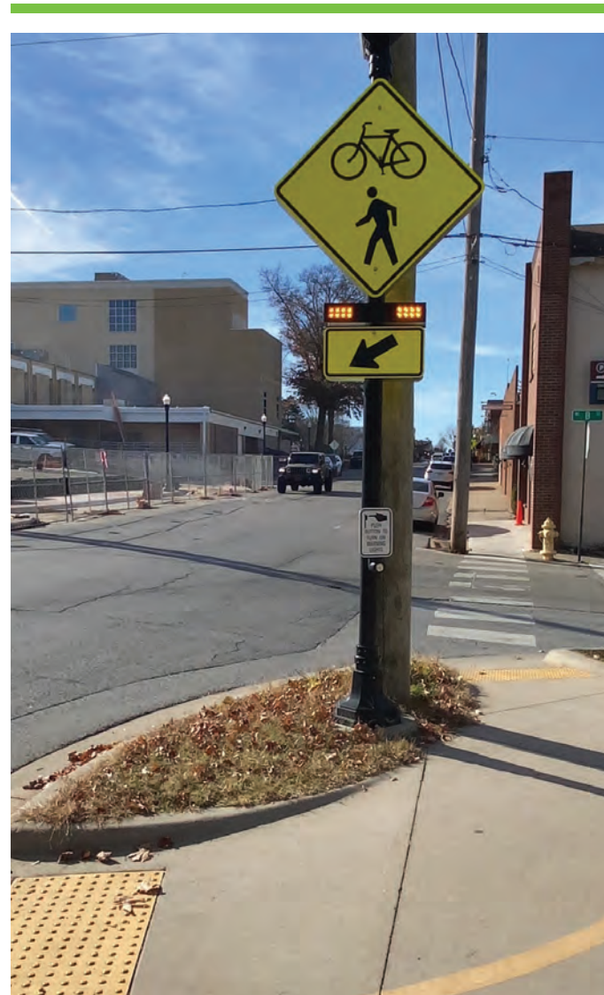
Multi-use trail safety features are designed for trail users and motorists. Traffic control signage should adhere to MUTCD guidance - particularly at locations where both parties will interact.
