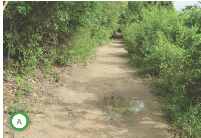
The gravel material and slope of the River Trail create drainage issues along the trail (A). Additionally, the surface material of the River Trail, limits trail users because of uneven surface and rock obstructions along the trail (C, D). However, the built structures along the trail, such as the restroom facilities (B) are in excellent condition and are accessible to all types of trail users.
