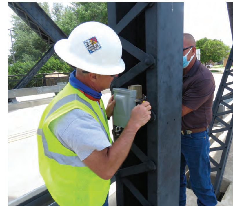
City staff installing trail and sidewalk counters as part of the master planning process.
