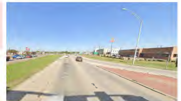
Existing Condition: SL-340 (Industrial Blvd) at Upper 13 Rd facing east
