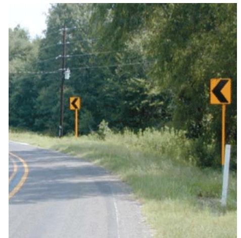
Chevron signs with retroreflective strips on sign posts installed along a curve. Source: FHWA
