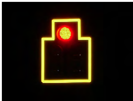
Retroreflective borders are highly visible during the night. Source: South Carolina DOT
