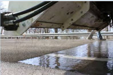
Automated application of HFST. Source: FHWA
