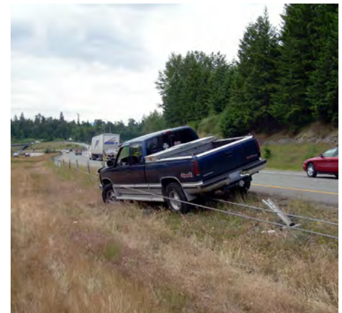
Median cable barrier prevents a potential head-on crash. Source: Washington State DOT
