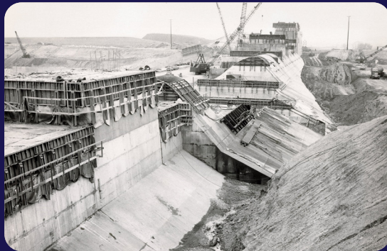
Construction of the Lake Waco Dam expansion in 1963. Photo courtesy of the Texas Collection.
