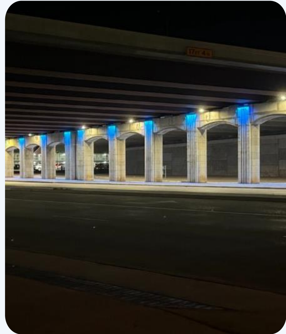
I-35 at Martin Luther King, Jr. Blvd. Underpass
